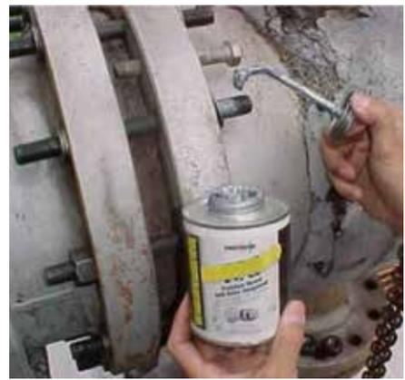
Fig. 8: Correct bolt lubrication.
