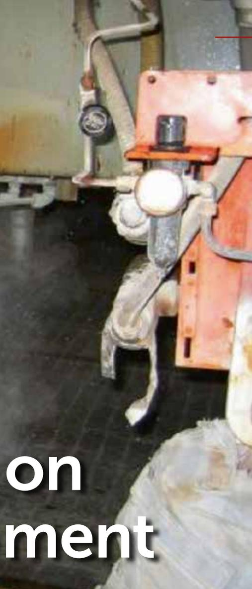
Fig. 1. Steam leaking from a valve.
