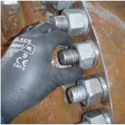
Fig. 7: The installation of flange Live Loading on a shell and tube heat exchanger.
