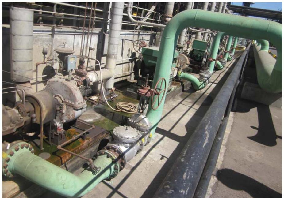
Cooling tower hard piped line before retrofit with rubber expansion joint
