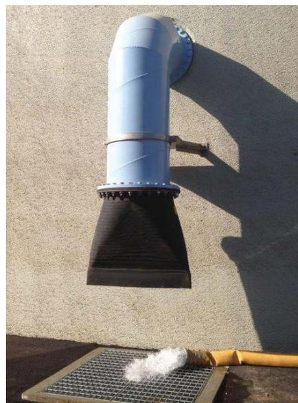
Duckbill check valve for tank overflow at water facility. Source images: Proco Products.
