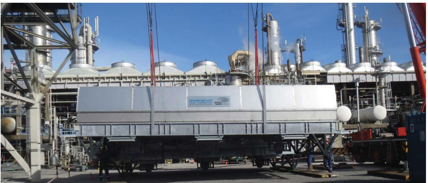
*Installation of complete cooler bundle adjusted with Whizz-Wheel*
