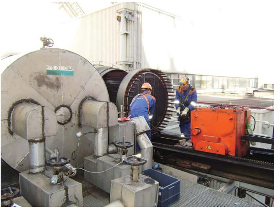
*Installation of bundle in heat exchanger*
