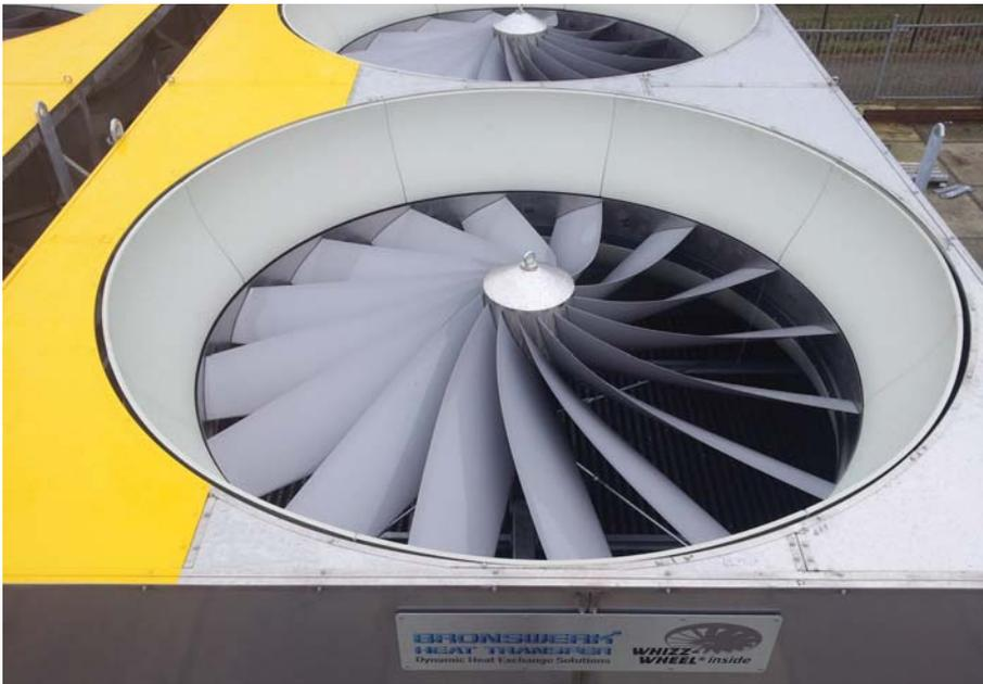
*Whizz-Wheel installed in cooler bundle to increase efficiency*
