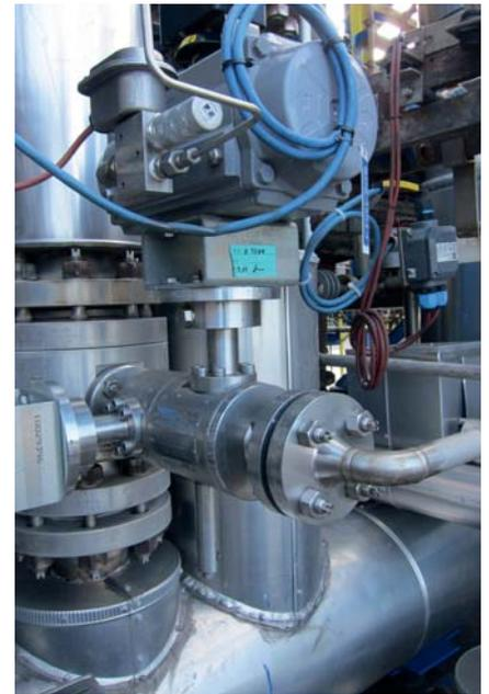
The four reactors of the POX-gasification plant at Yara Brunsbüttel with their gastight and metal-to-metal sealing ball valves - a customized Hartmann design for high temperatures, steam and pure oxygen.
