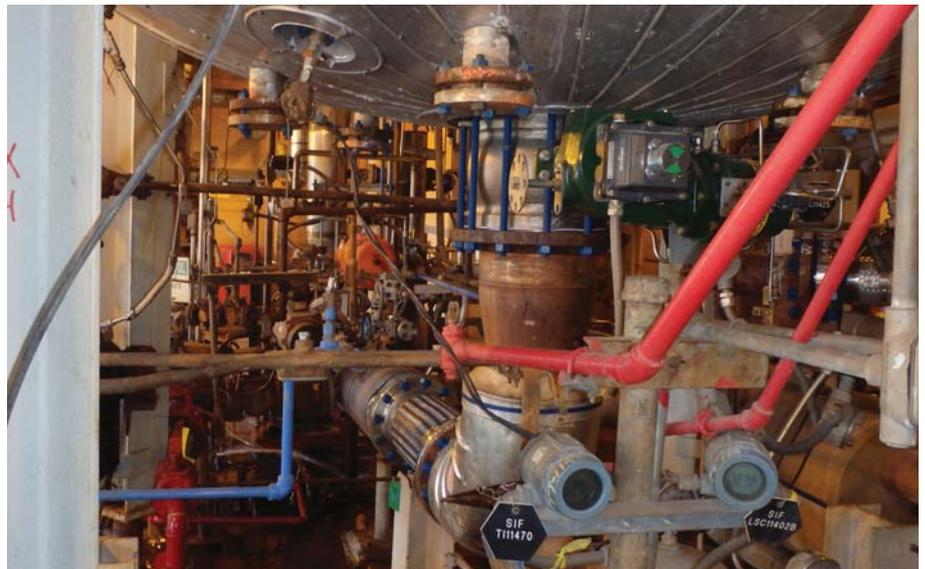
*The insulated hemispherical head of the reactor is shown installed with a hose to accommodate the downward thermal growth on a line connected to a pump. The hose protects the pump as well as improves the performance of the weight cells on the reactor.*
